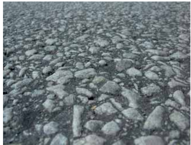
Thin layer surface from Ellenborgsvägen in Malmo Photo: Danish Road Institute
