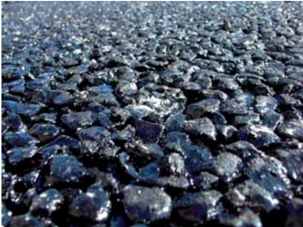
Porous asphalt from Lyngbyvej in Copenhagen
